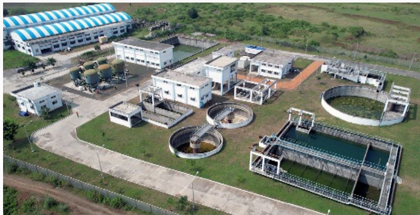
Sewage Treatment Plant
